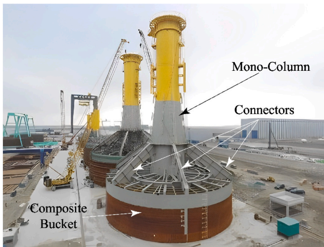
Fig. 1. Photograph of the MCCBF (a large-diameter Mono-Column Composite Bucket Foundation with six connectors).
